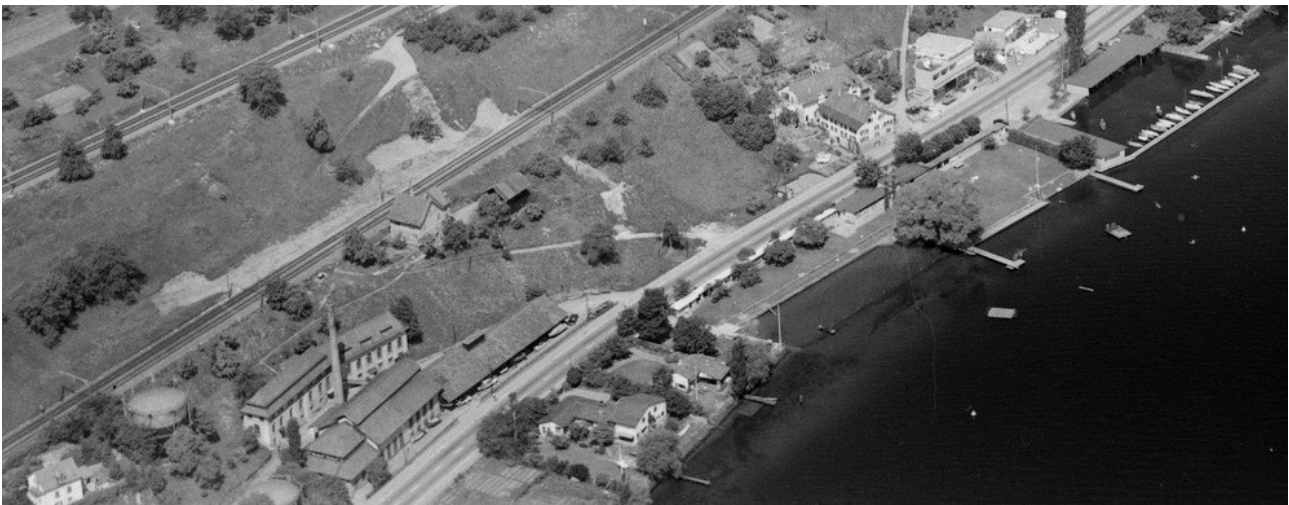
Circa 1962 Lower left is the gasworks
